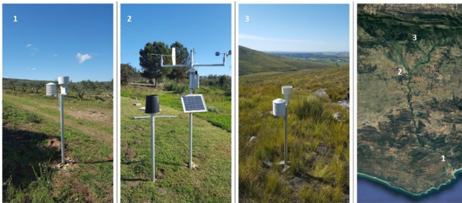
Figure 11: Three weather stations were installed to capture data for hydrological modelling.
